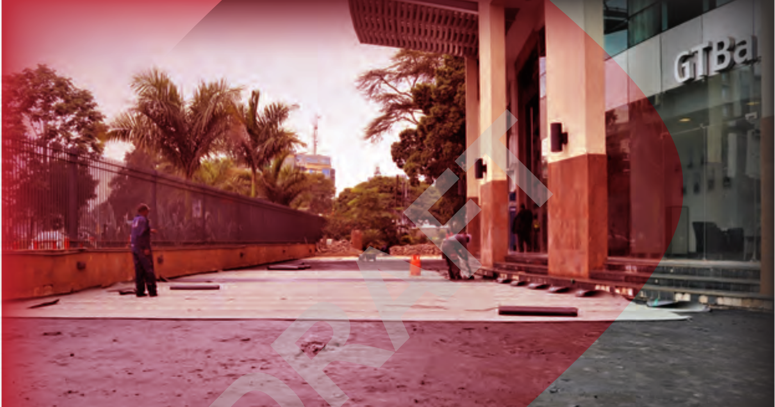
Laying of App Waterproof Membrane at parking area, to protect the base- ment parking beneath at Skypark Building in Westlands.
